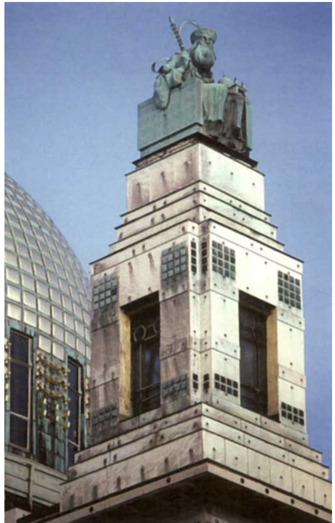
8 Steinhofkirche, detail of roof figure of Saint Severin, designed by Richard Luksch, view of 2002 (photo: Michael Wabb)
