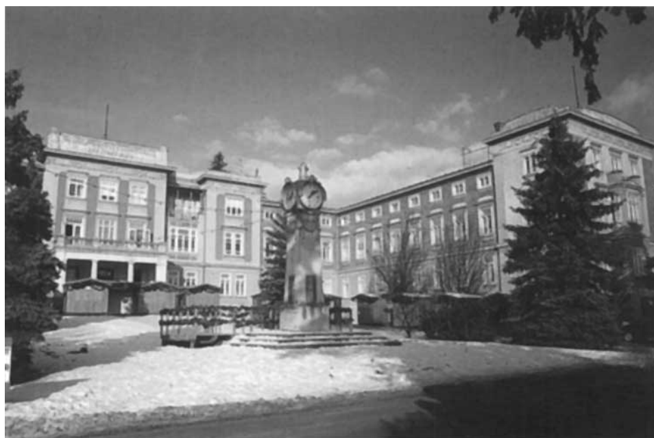
3 Franz Berger, administration building, Steinhof, 1903–7, view of 2002 (photo: Michael Wabb)
